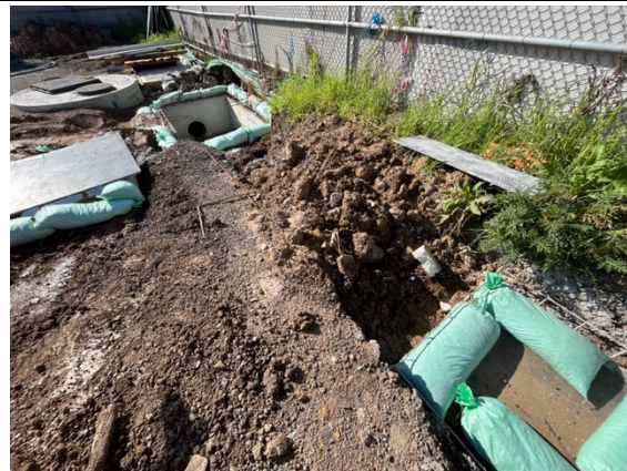
Photos 11 - 14: Erosion and sediment controls in place including rumble grid at heavy vehicle access (Photo 1). Sediment fencing installed along the Schofields Road southern boundary, and controls around new stormwater infrastructure (not yet connected) in place. Sediment fence requires repair in one location due to water ingress from Schofields Road.
