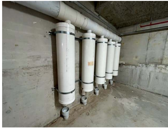
Photo 7: Site 1 – First flush system for the reuse of greywater in the future retail space
