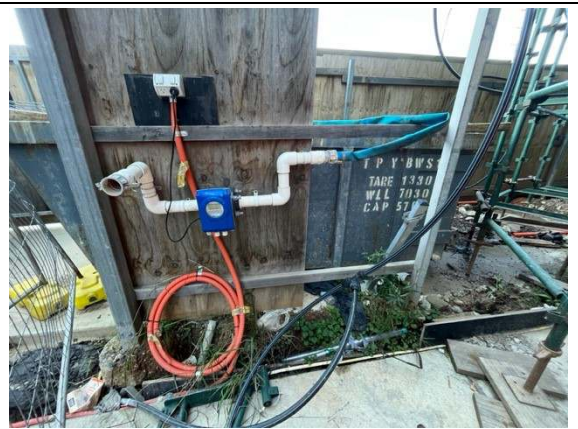
Photos 5 & 6: Site 1 – Basement carpark groundwater collection point and sediment tank on Ground level with flow meter in place
