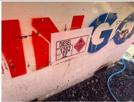
Photos 8 & 9: Hazardous chemical storage in bunded and labelled containers. A spill kit needs to be provided near the diesel storage area
